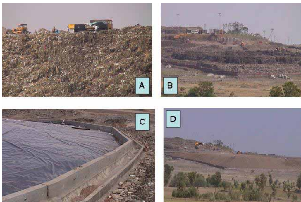
A – Dumpsite; B – Work in progress; C – Cover and storm drains; D – After reclamation
